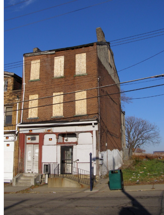
August Wilson's Birthplace, Bedford Avenue, The Hill District, Pittsburgh, PA
